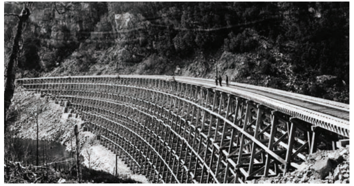
FIGURE 5-33 This wooden railway trestle, 33 m high and 270 m long, is in Ontario. Look closely at the landscape and the scale of the bridge. Even though it was the cheaper option, what kind of time and resources would have been spent to build this bridge? How many wooden bridges do you think were built across Canada?
